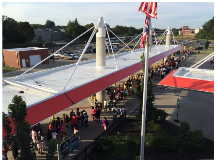
Over 3,000 customers use the Robert K. Pfaff Intermodal Transportation Center each weekday. The heart of METRO's network, RKPTC also berths Greyhound, ODOT GO rural transit, PARTA and SARTA buses. Opened in 2009, it earned a LEED Gold Certification. Shown are "I Promise" program participants preparing to board 65 coaches chartered by the LeBron James Family Foundation for its 2015 Family Reunion at Cedar Point.
