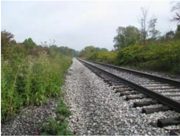
Photo 18: Track Section (looking north)
