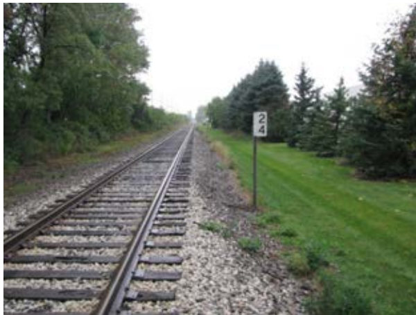
Photo 12: MP 24 (looking south)
