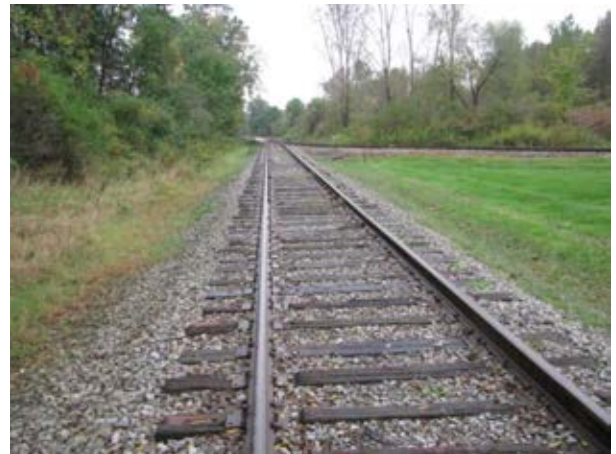
Photo 15: Track Section (looking south)
