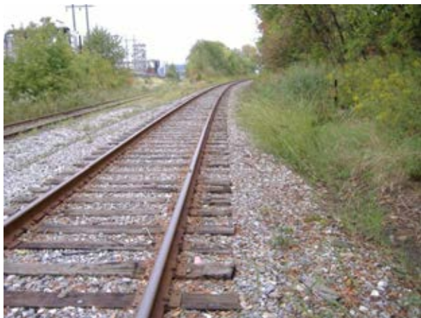
Photo 31: Track Section (looking south)
