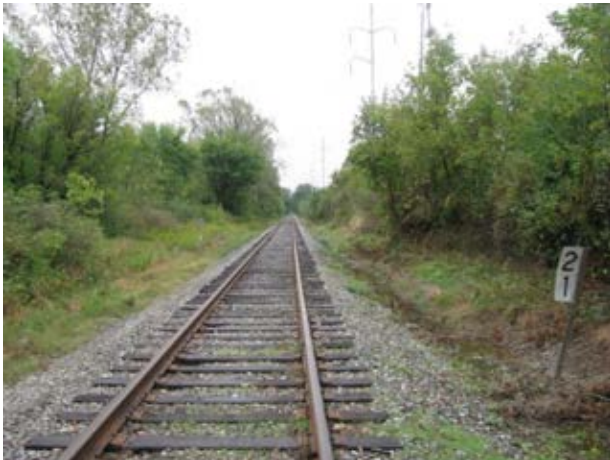
Photo 6: MP 21 (looking south)
