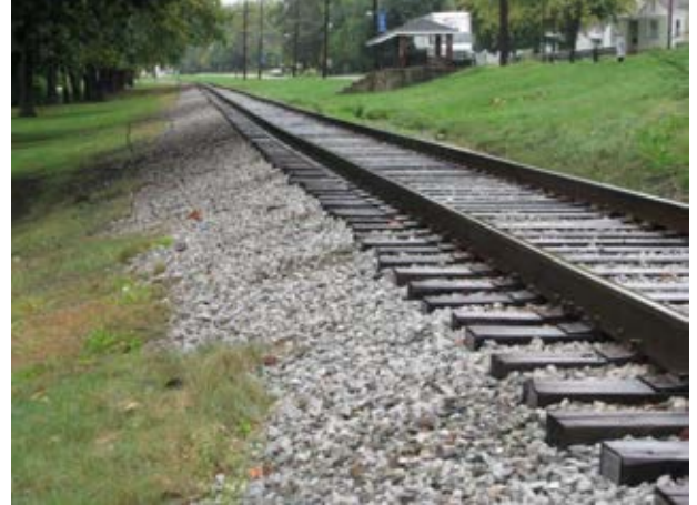
Photo 3: Track Section (looking north)
