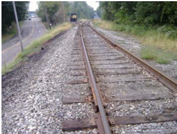
Photo 36: Track Section (looking north)
