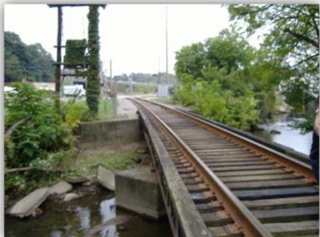
Bridge 431 looking south towards Case Avenue along the Sandyville Line.
