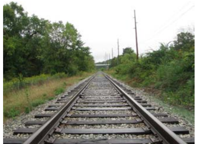
Photo 4: Malone Parkway Overpass (looking north)
