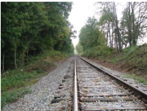
Photo 19: Track Section (looking south)
