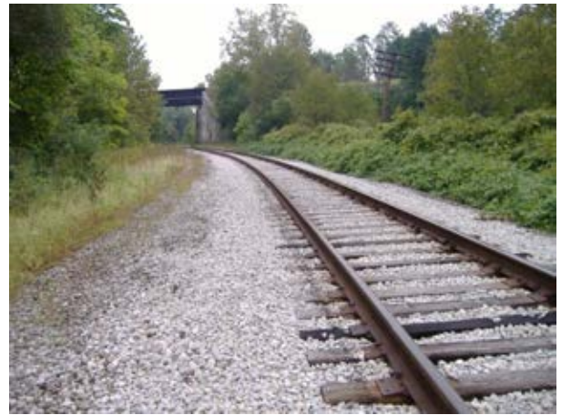
Photo 33: Track Section (looking north)
