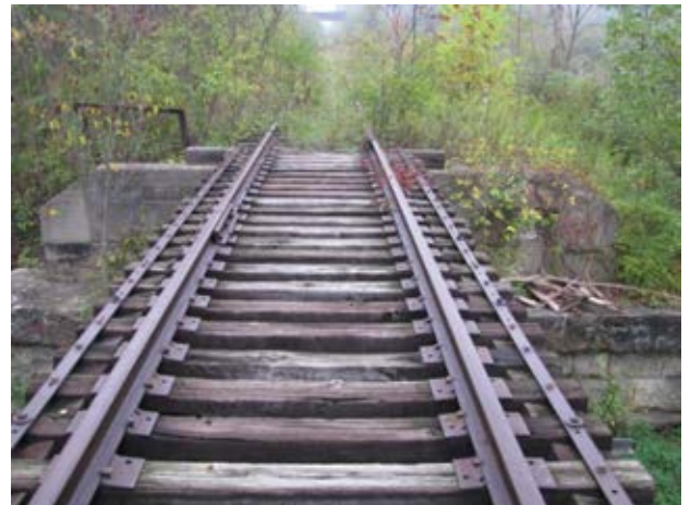
Photo 4: Structure over Powers Creek
