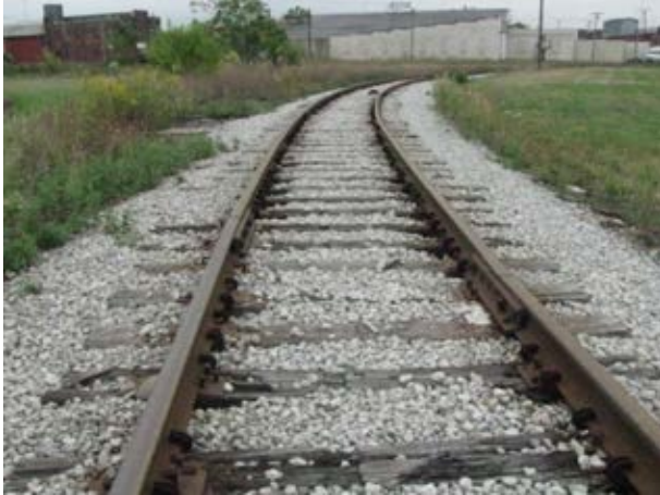
Photo 1: Curve (looking south)
