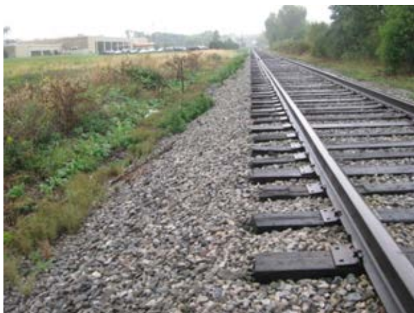
Photo 13: Track Section (looking north)
