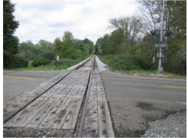
Photo 20: MP 28 Heckman Road (looking north)
