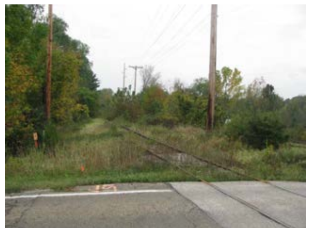
Photo 6: Barlow Road crossing surface (looking south)
