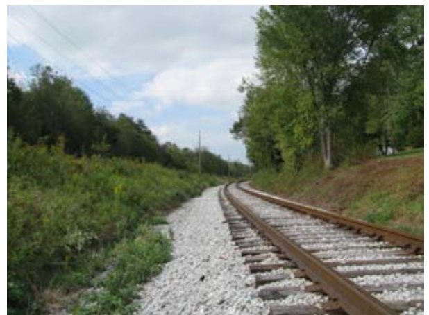
Photo 28: Track Section (looking north)
