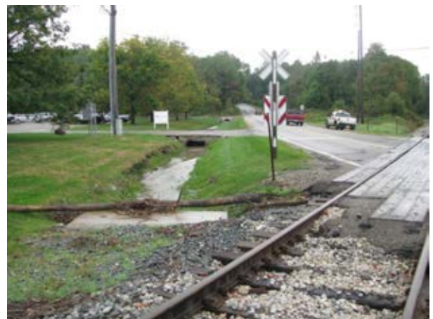
Photo 16: Culverts (looking northwest)
