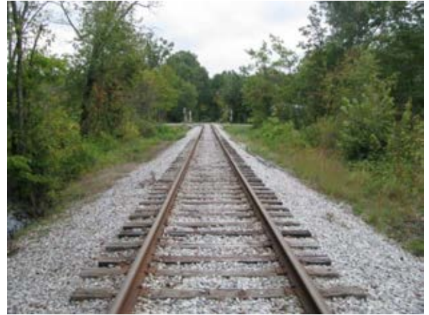
Photo 26: Track Section (looking south)
