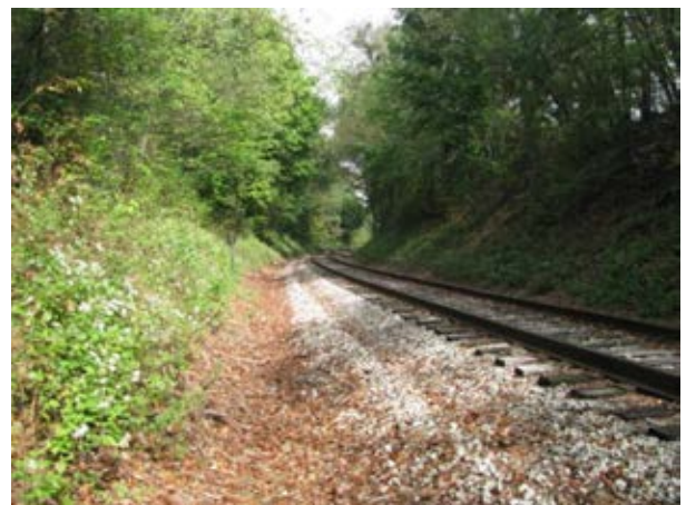
Photo 22: Track Section (looking north)
