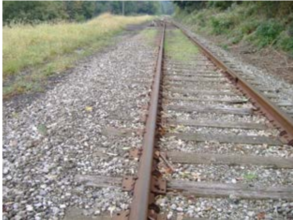
Photo 35: Track Section (looking south)
