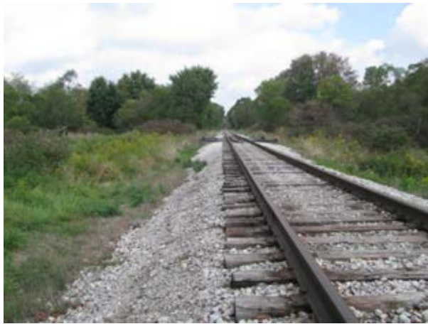
Photo 24: Bridge 427 (looking north)
