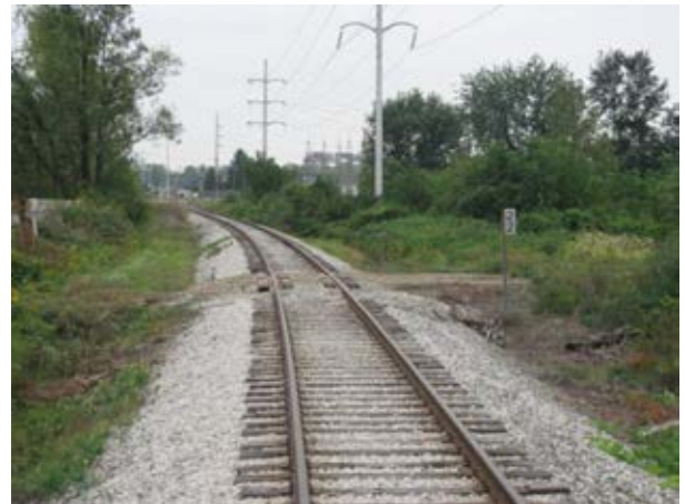
Photo 9: MP 22 (looking south)
