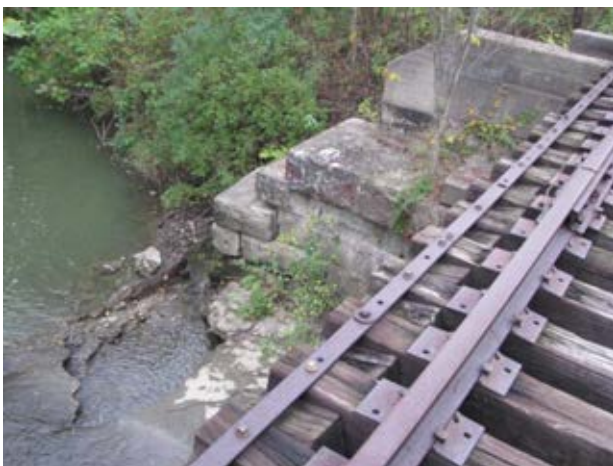
Photo 5: Structure over Powers Creek (northwest wingwall)
