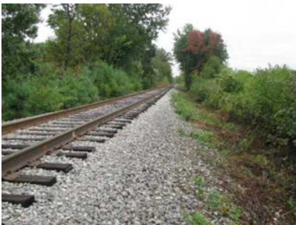
Photo 7: Track Section (looking south)
