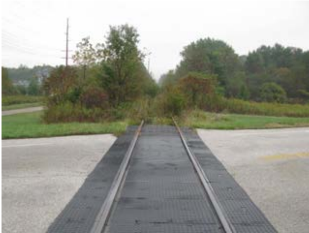
Photo 1: Seasons Road at-grade crossing surface (looking north)
