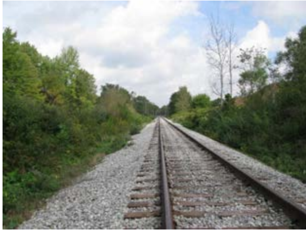
Photo 23: Track Section (looking north)
