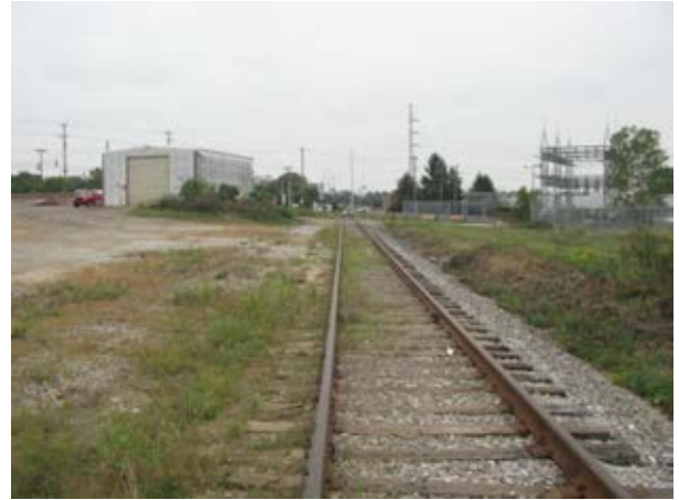
Photo 8: N of Whipple St. (looking south)
