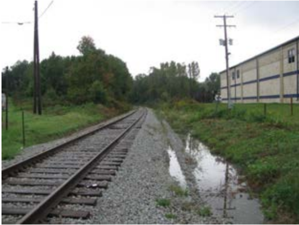
Photo 17: Track Section (looking north)
