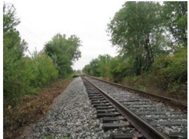
Photo 10: Bridge 423 (looking north)
