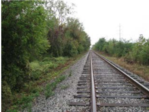
Photo 11: Track Section (looking south)
