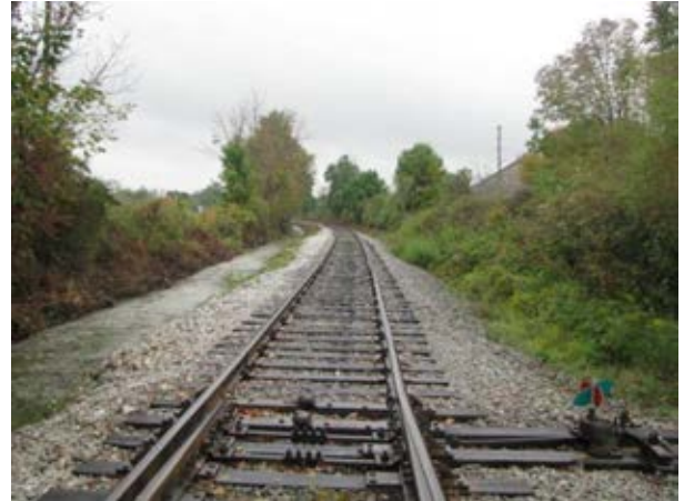
Photo 14: Track Section (looking south)
