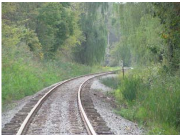
Photo 25: MP 30 (looking south)
