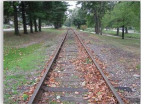
View along the Sandyville Line
