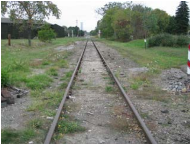
Photo 2: Buried Ties (looking north)
