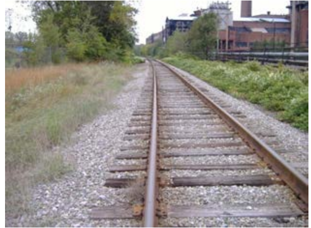
Photo 32: Track Section (looking north)
