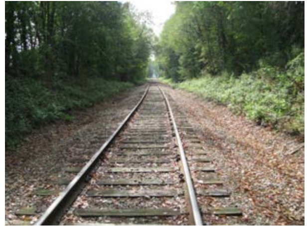
Photo 21: Track Section (looking south)
